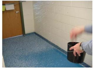
For the most uniformed appearance many contractors like the "Total Broadcast". This is done by taking small hands full of the chips and broadcasting them into the floor.
